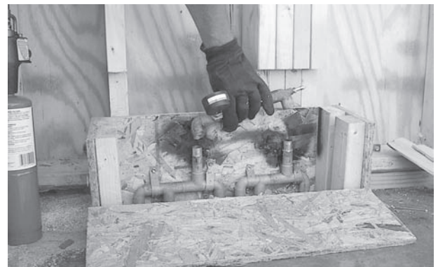
Removing the pressure testing assembly
