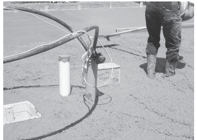
Pouring the slab around the manifold box
