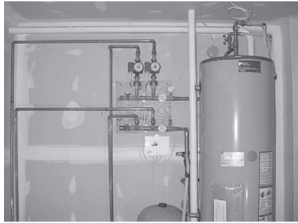
A two zone open system. 2" PVC is used for exhaust. No chimney is required.
