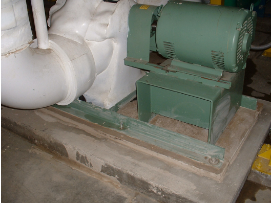
Figure 8 - Typical pump base grouting
