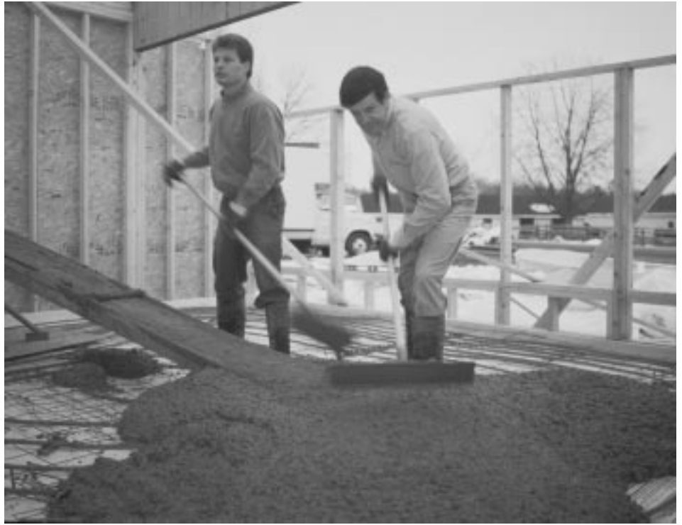
Fig. 5.21: Tube is pressurized during thermal mass installation.
