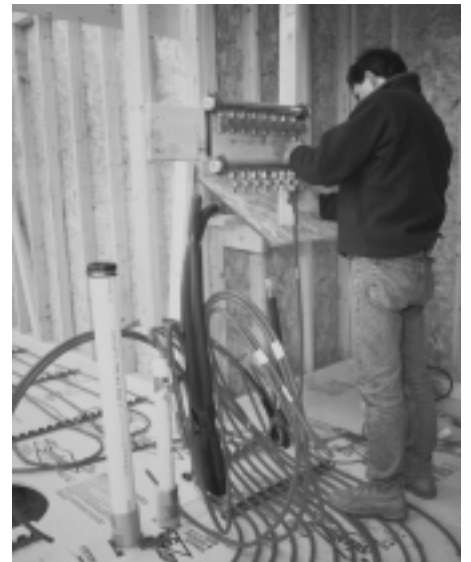
Fig. 5.19: Manifold to tube connection.
