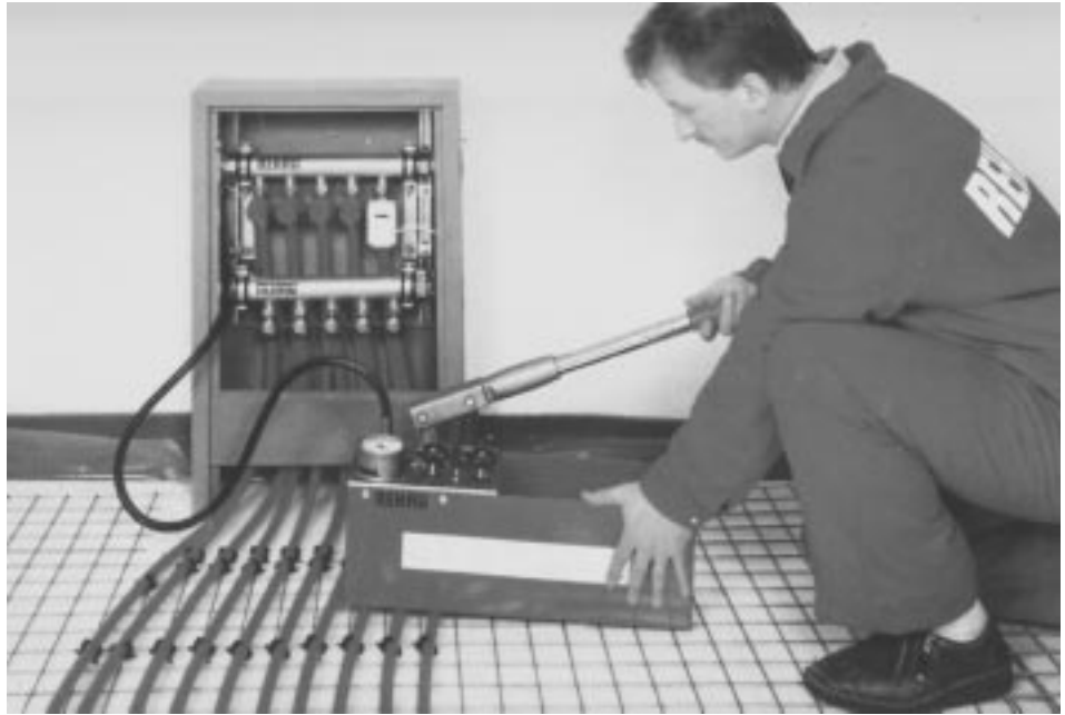
Fig. 5.20: Pressure tests.
