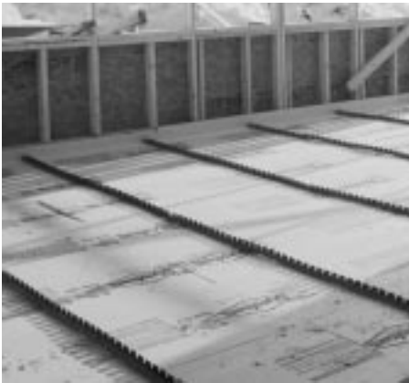
Fig. 5.9: RailFix with 3' (1 m) spacing ready for tube.
