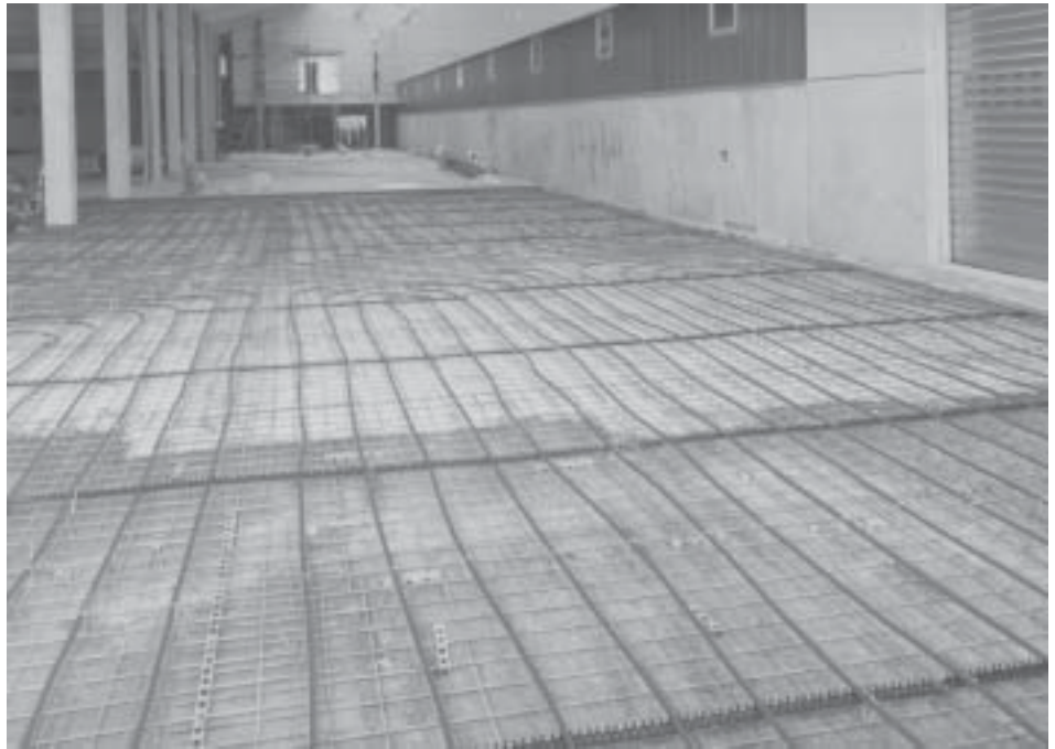
Fig. 3.1: REHAU underfloor heating.
