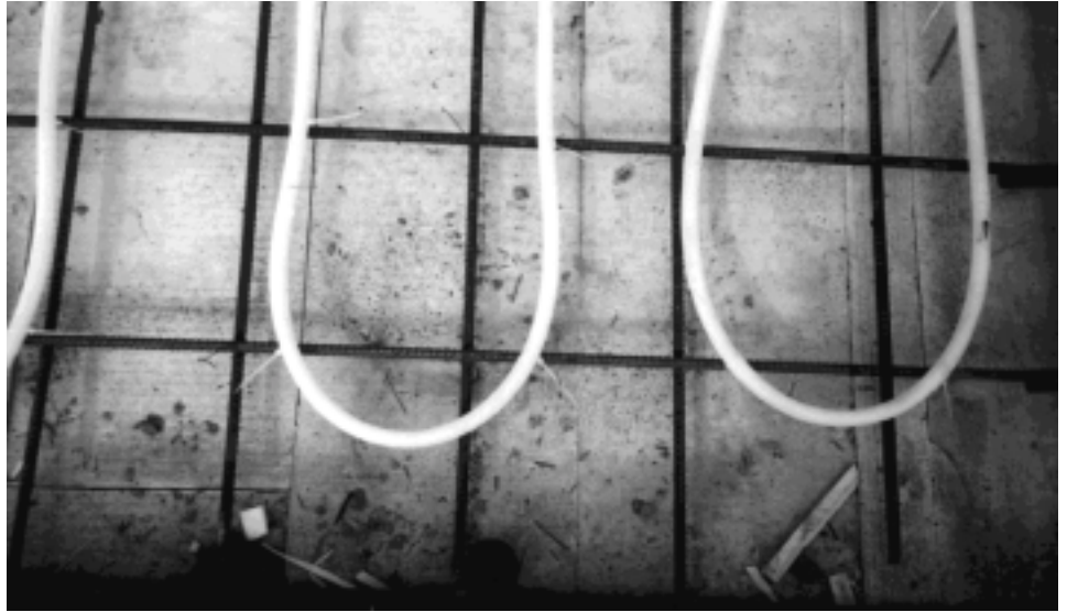
Fig. 5.4: Cable binder method with rebar.
