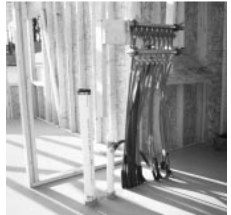
Fig. 5.23: Protection sleeves at slab penetrations.
