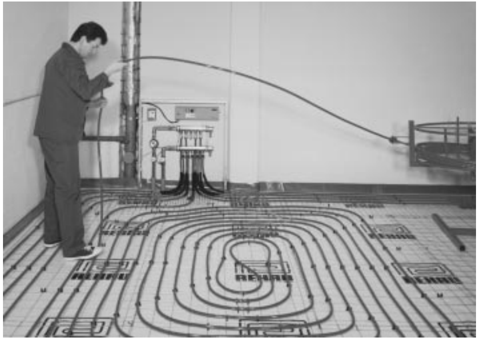
Fig. 5.18: Tube and manifold installation.
