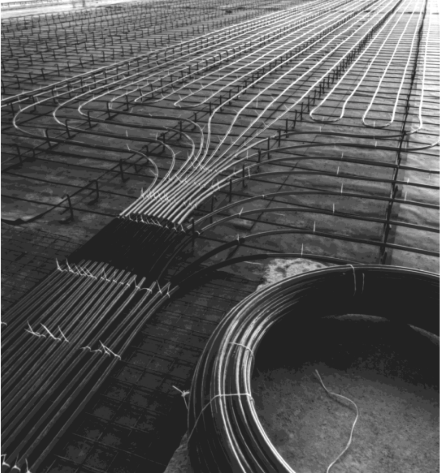
Fig. 2.1: REHAU system using 25 x 2.3 RFH tube and cable binder method of installation.
