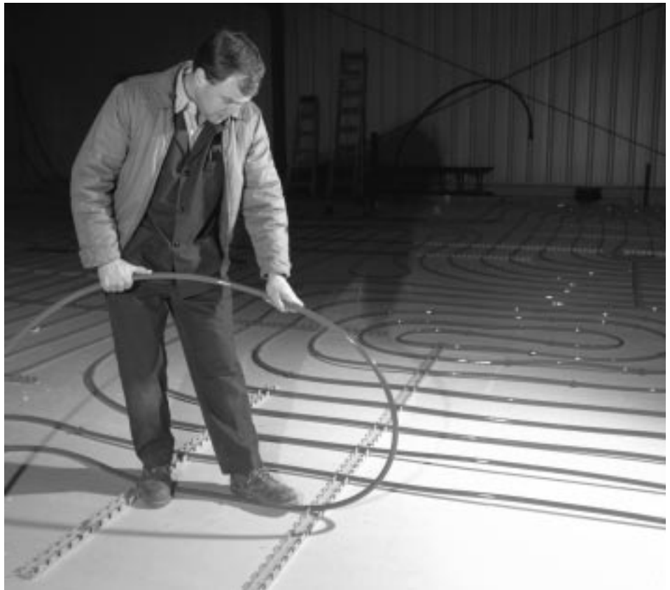
Fig. 5.10: Layout tube in accordance with design plans.
