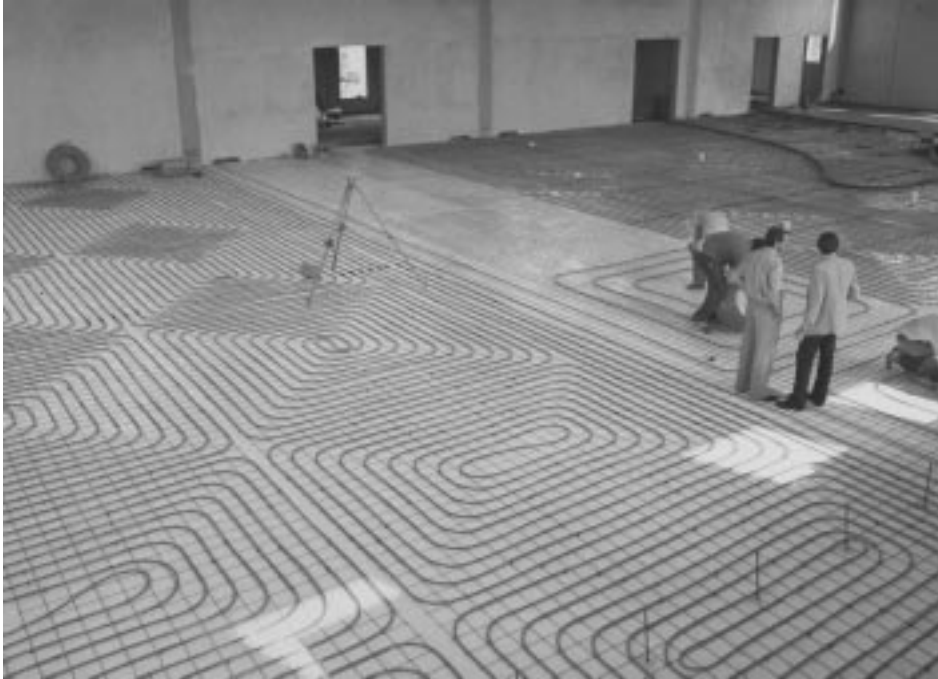
Fig. 1.1: REHAU radiant floor heating in an industrial project.
