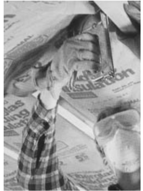
Fig. 5.12: Blanket insulation for joist space method.
